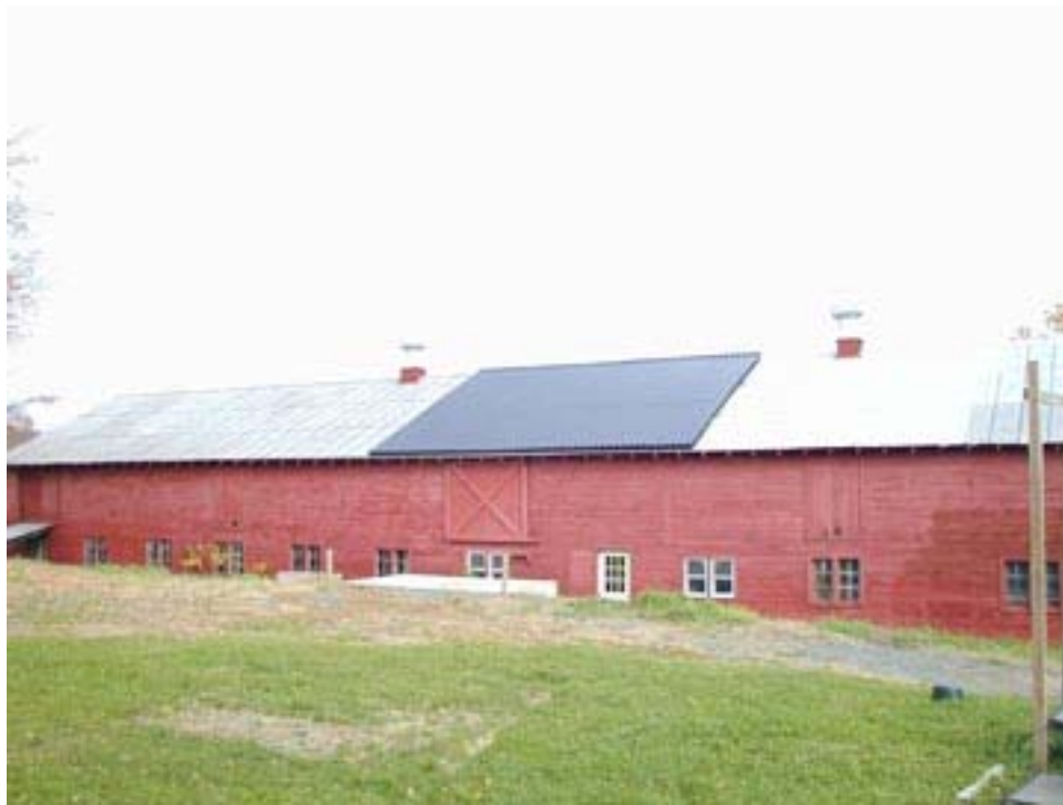
Figure 2. Solar panels on roof of barn, which increase the temperature in the loft, helping to dry wet wool and to heat the downstairs production area in winter.
